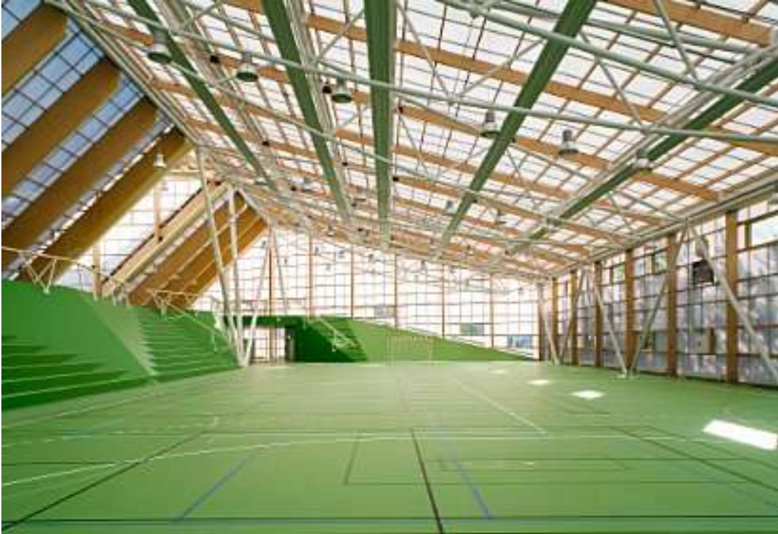
Competition Venue Holmbladsgade 71 – 2300 Copenhagen, Denmark
